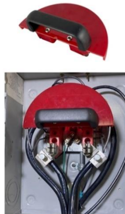
Figure 18 – Protection From Energized Parts.
