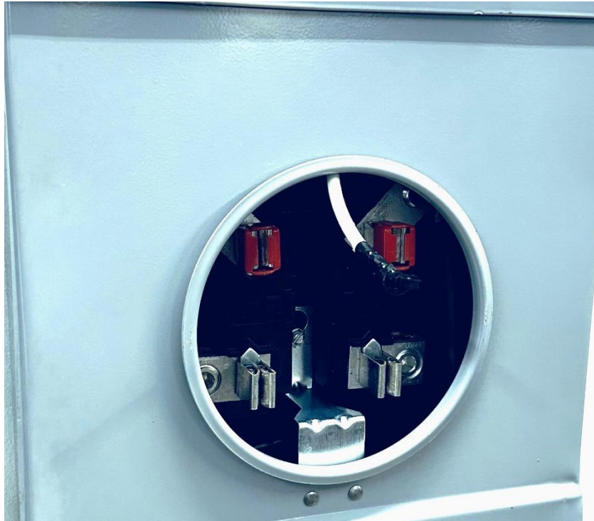
Figure 24 – Reinstall the Ring-Type Cover.
