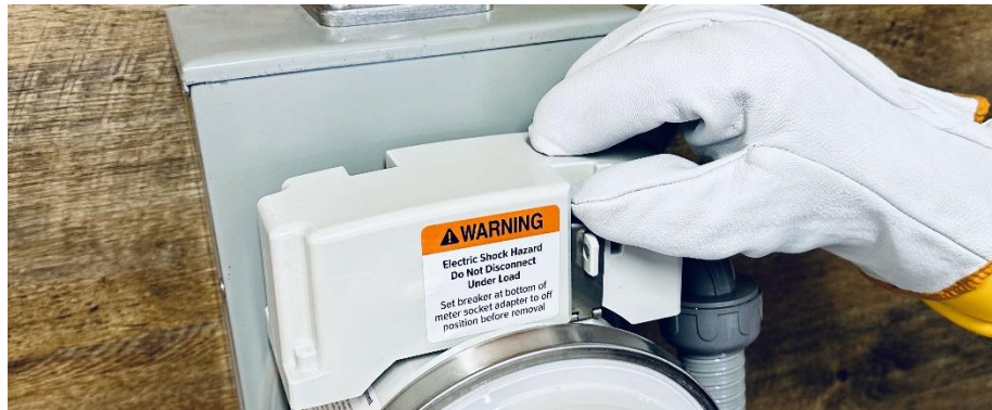
Figure 40 – Secure the Connection Module Clasps.
