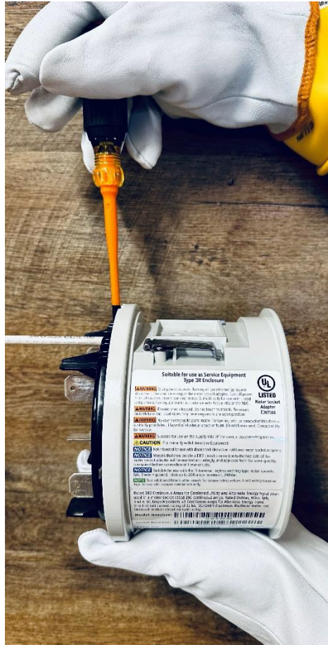
Figure 27 – Terminate the Neutral to the Solar MSA Base.
