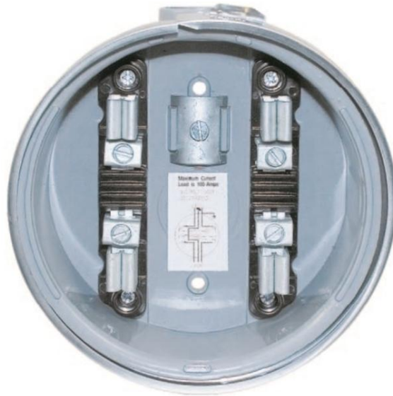
Figure 4 – Shallow Meter Socket (not recommended).
