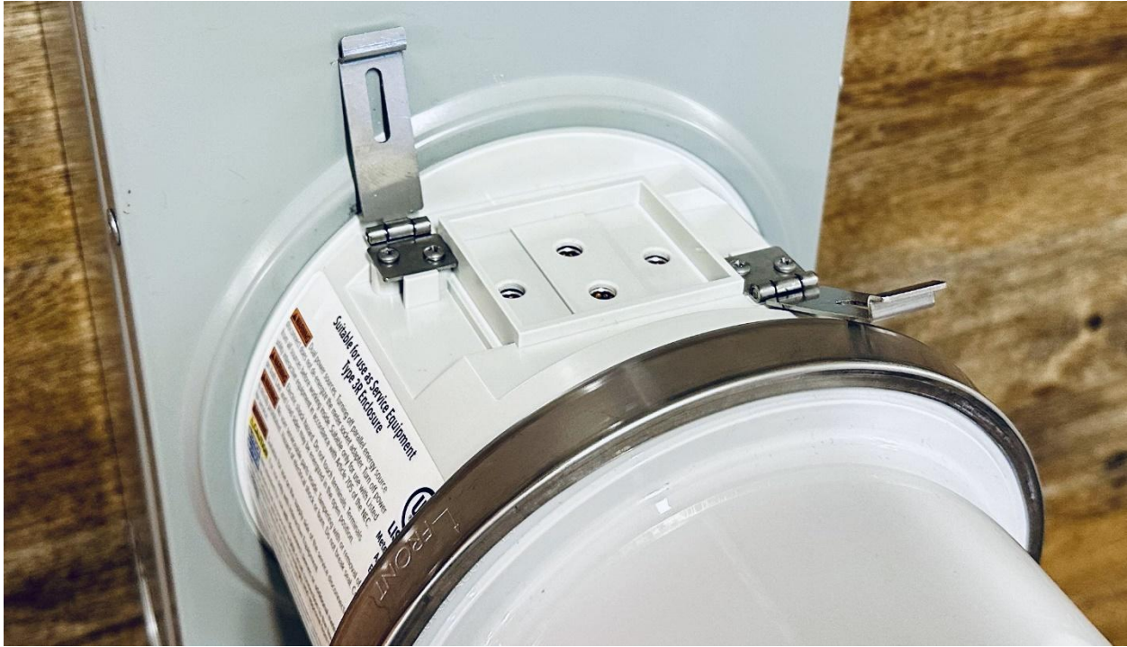
Figure 32 – Connection Module Clasps.
