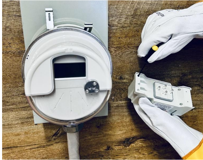
Figure 36 – Connection Module Removed from the MSA Base.
