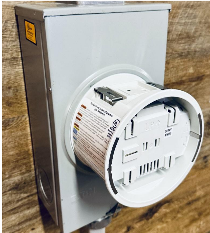
Figure 29 – Reinstall the Meter Socket Cover.
