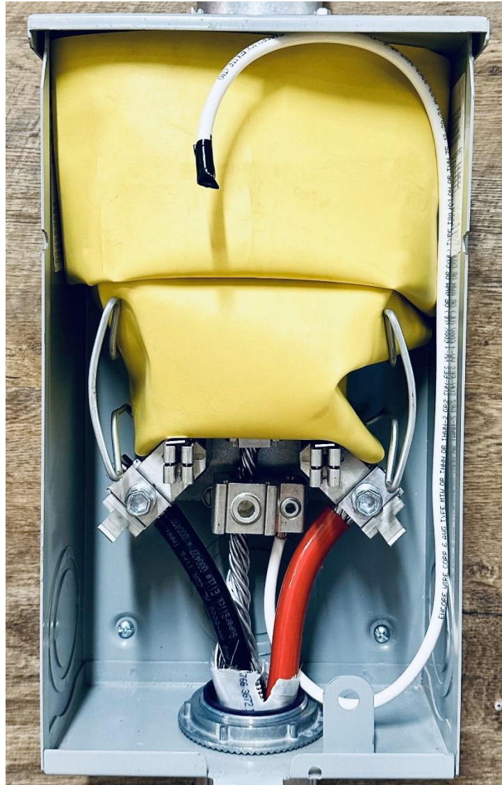
Figure 23 – Route the Neutral Within Meter Socket.
