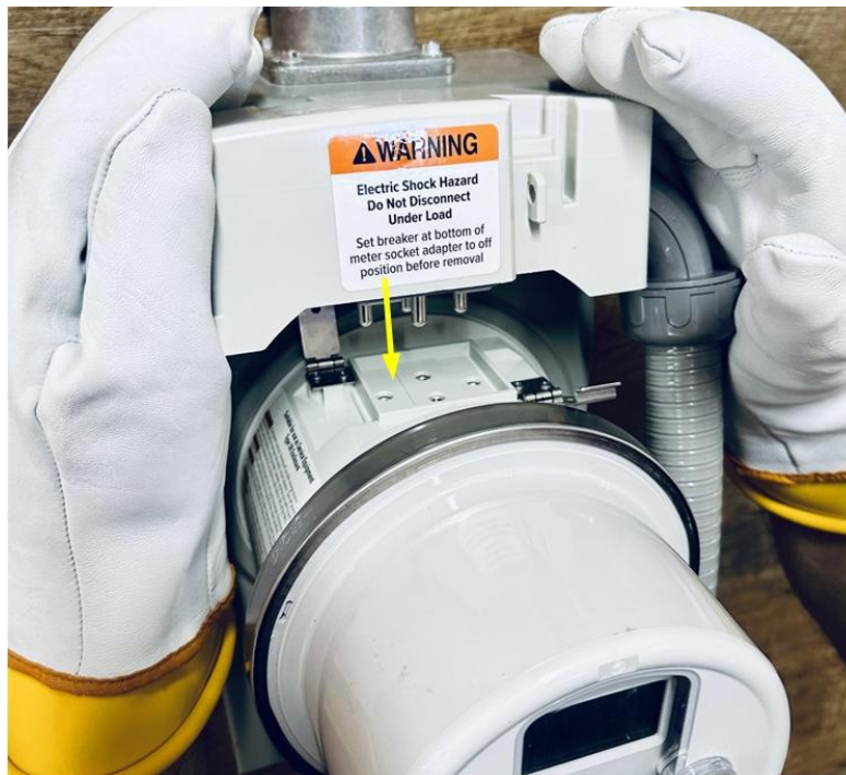
Figure 39 – Align the Connection Module Pins over the Power Interface of the MSA Base.
