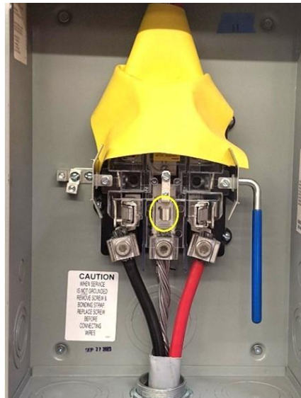
Figure 16. Protection From Energized Parts.
