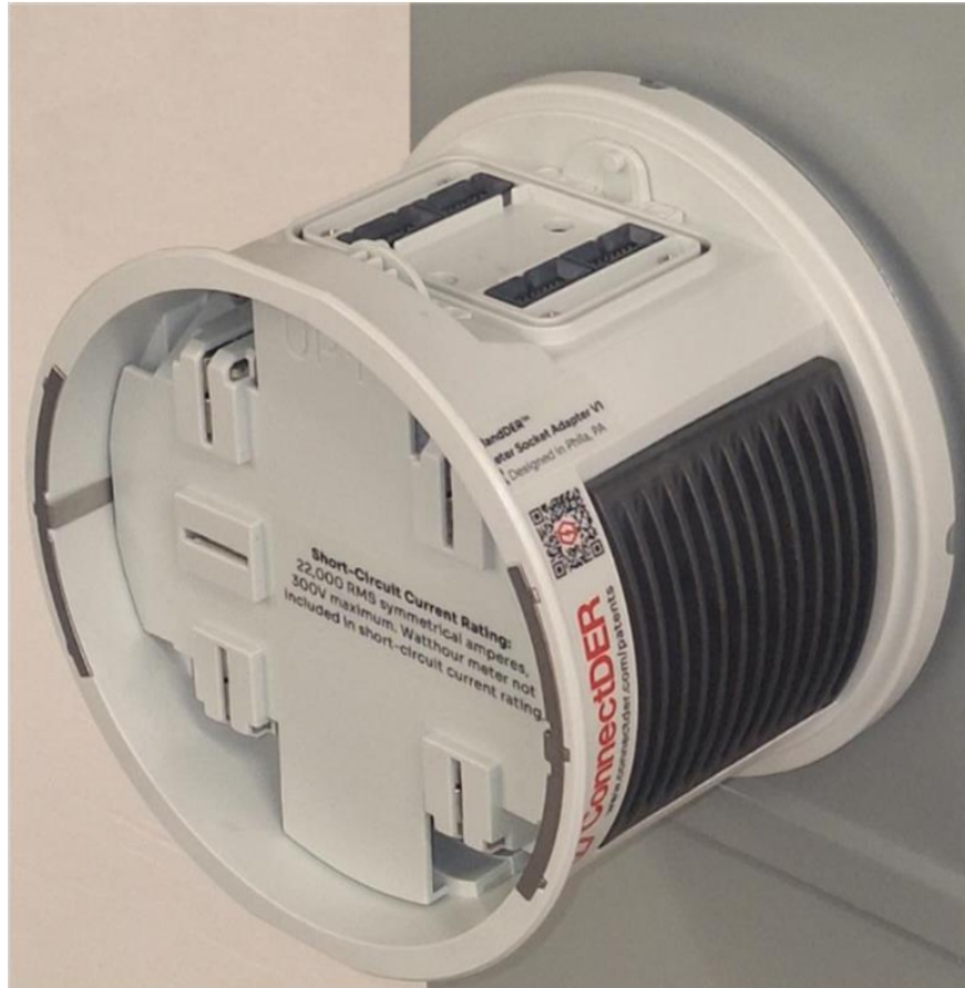
Figure 21. MSA Base Inserted in ringless socket.
