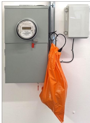
Figure 45. DER System Completed, Ready for MSA Installation.
