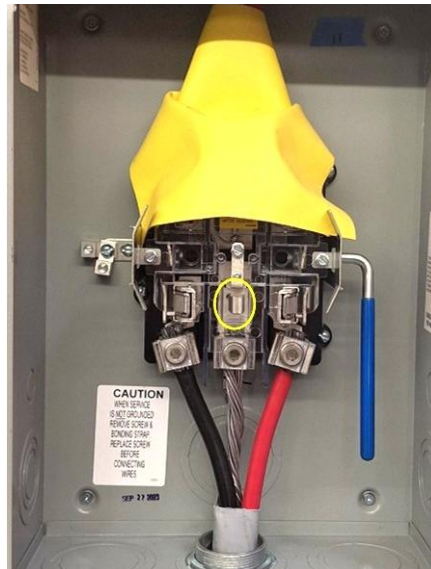
Figure 16 – Protection From Energized Parts.
