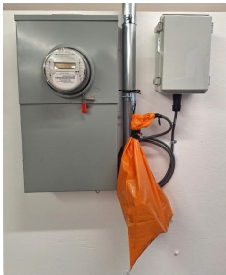
Figure 42 – DER System Completed, Ready for MSA Installation
