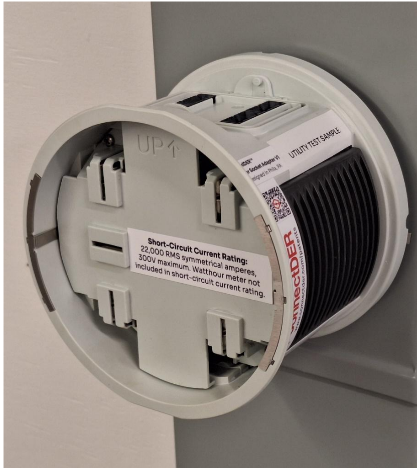
Figure 21 – MSA Base Inserted.
