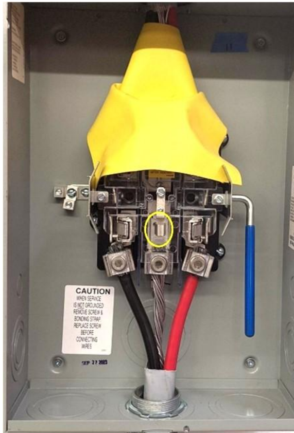
Figure 19 – Meter socket with 5 th jaw at 6 o'clock.
