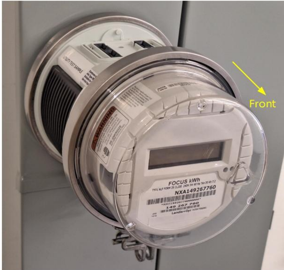
Figure 23 – MSA Base with Utility Meter Installed.
