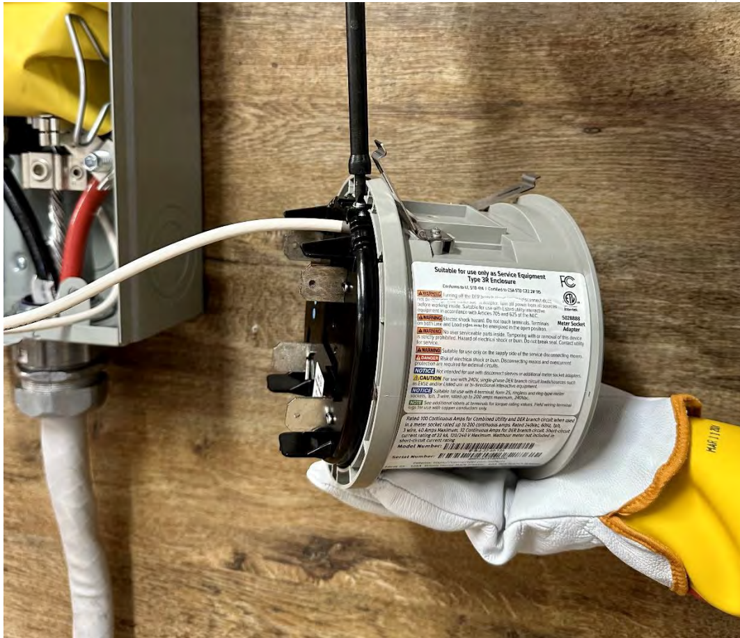
Figure 18 – Terminate the Neutral to the EV MSA
