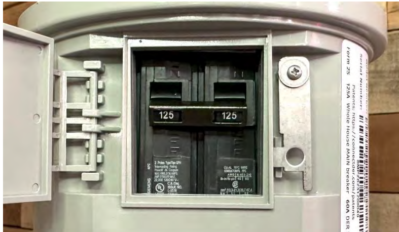
Figure 19 – Verify the whole-house MAIN circuit breaker is open (OFF)
