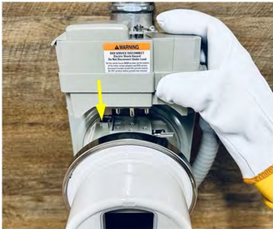
Figure 34 – Align the Connection Module Pins
