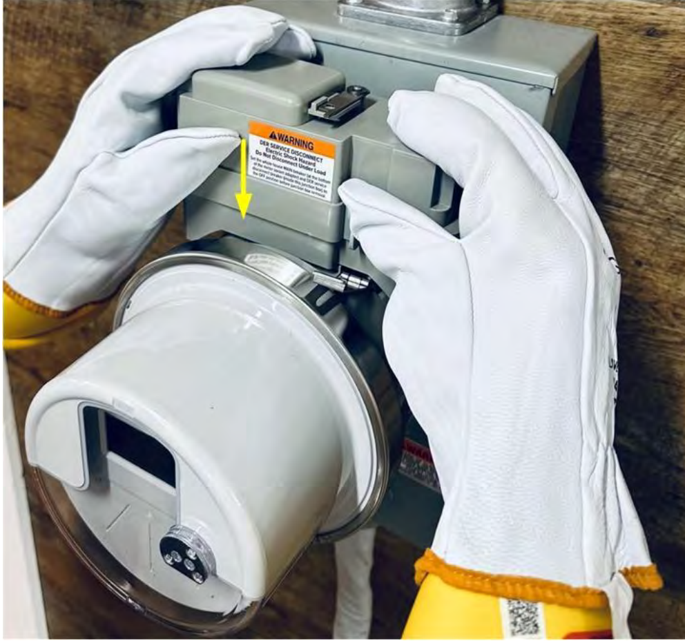
Figure 28 – Connection Module Installation
