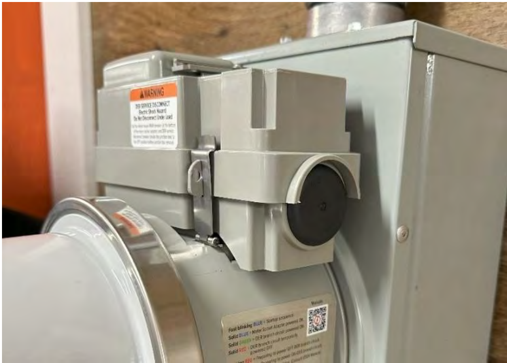
Figure 29 – Sealed Connection Module
