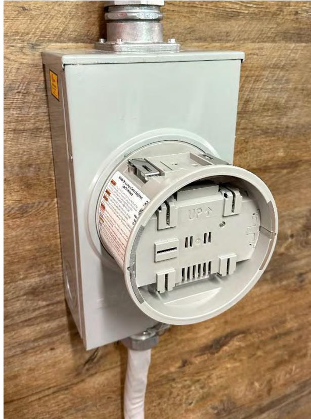
Figure 20 – Reinstall the Meter Socket Cover
