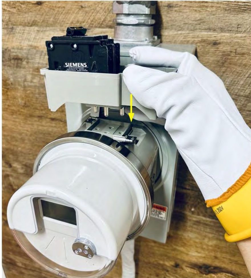
Figure 23 – Insert Connection Module Base
