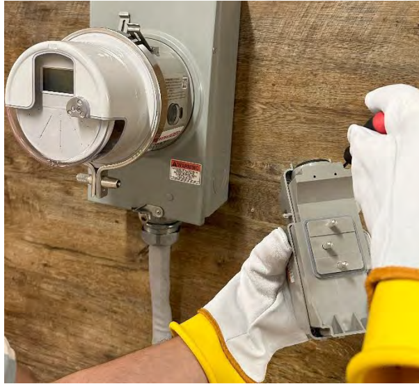
Figure 31 – Connection Module Removed.
