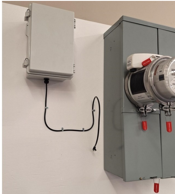
Figure 39 – Ethernet Cable in 3 rd Party Enclosure.
