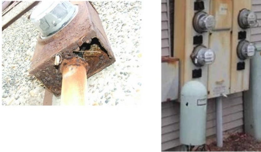
Figure 13 – Rusty, Damaged, Poorly-Mounted Meter Sockets.
