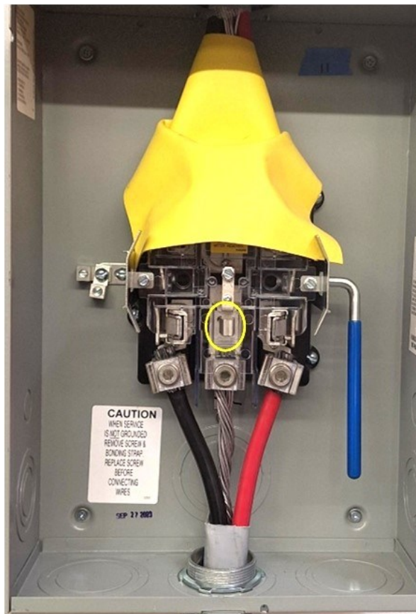
Figure 20 – Meter socket with 5 th jaw at 6 o'clock.
