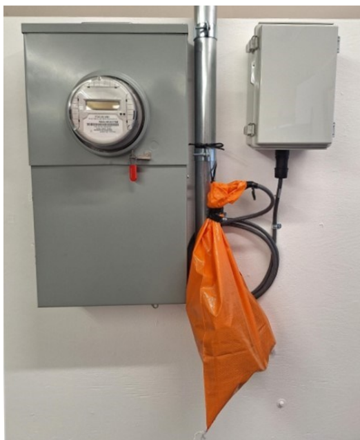
Figure 55 – DER System Completed, Ready for MSA Installation
