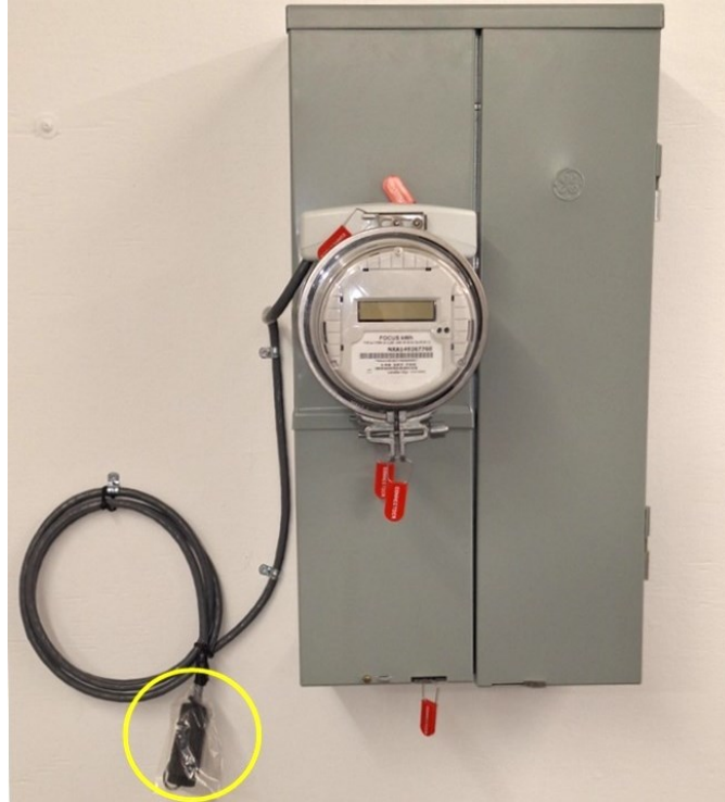
Figure 29 – IslandDER Analog Installed and Ready for 3 rd Party Integration.
