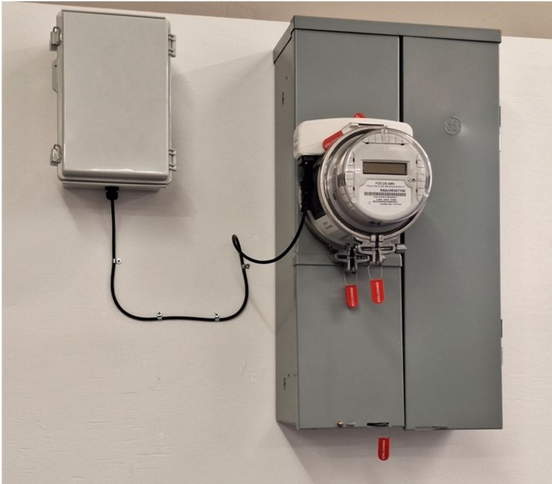
Figure 49 – IslandDER Digital MSA Complete to 3 rd Party System.
