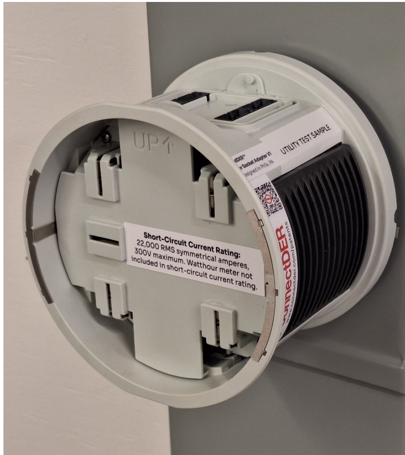
Figure 22 – MSA Base Inserted.
