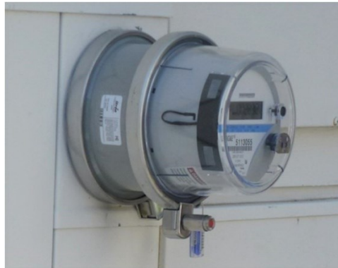
Figure 12 – Existing Meter and Meter Socket Adapter.
