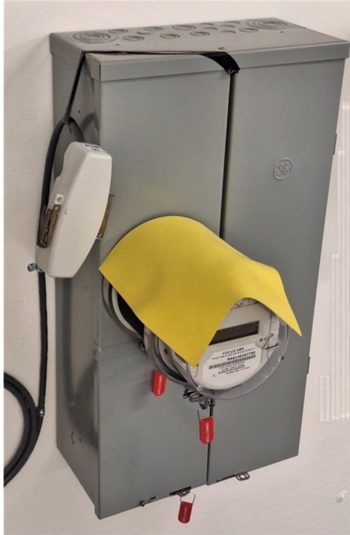
Figure 31 - Analog Connection Module Temporarily Supported, Communications Cable Deenergized, MSA Base Protected.
