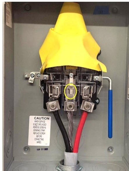
Figure 17 – Protection From Energized Parts.
