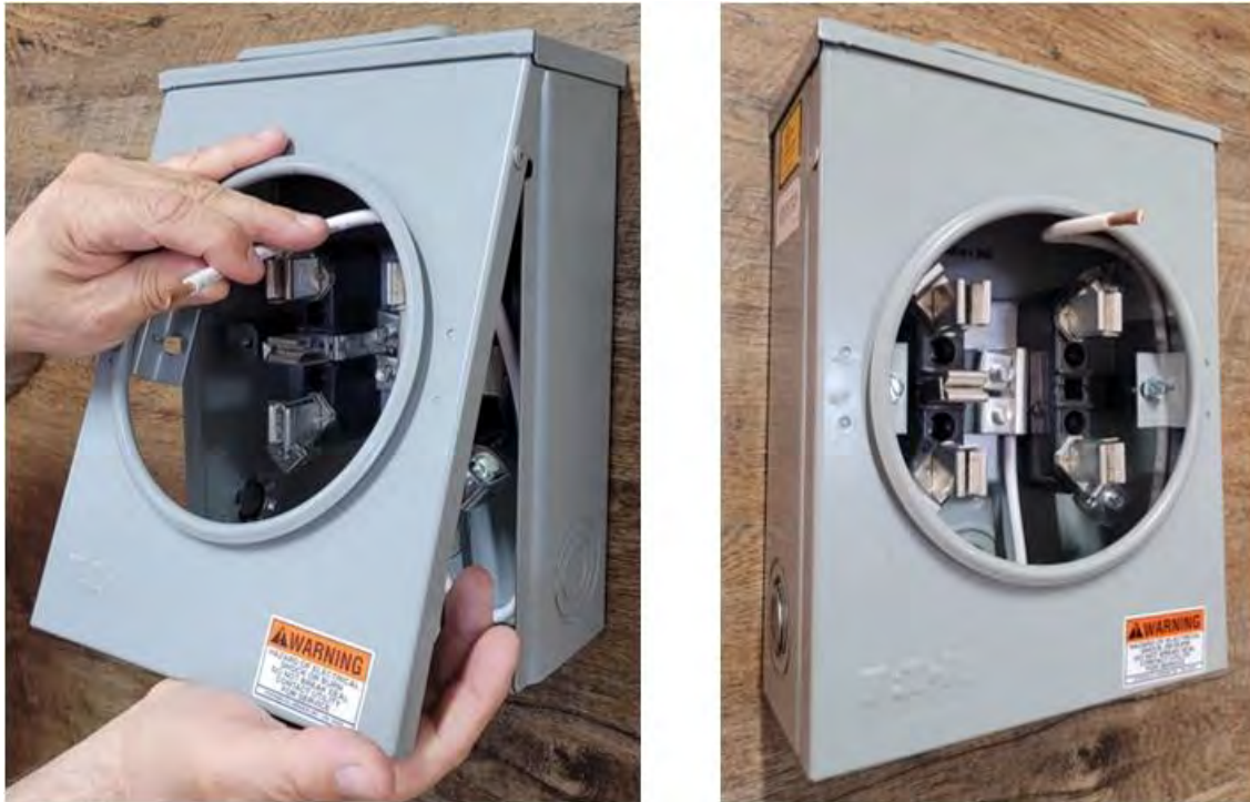
Figure 16 – Reinstall the Ring-Type Cover
