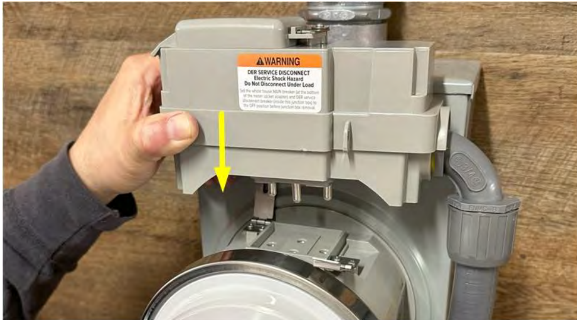
Figure 33 – Align the Junction Box Pins
