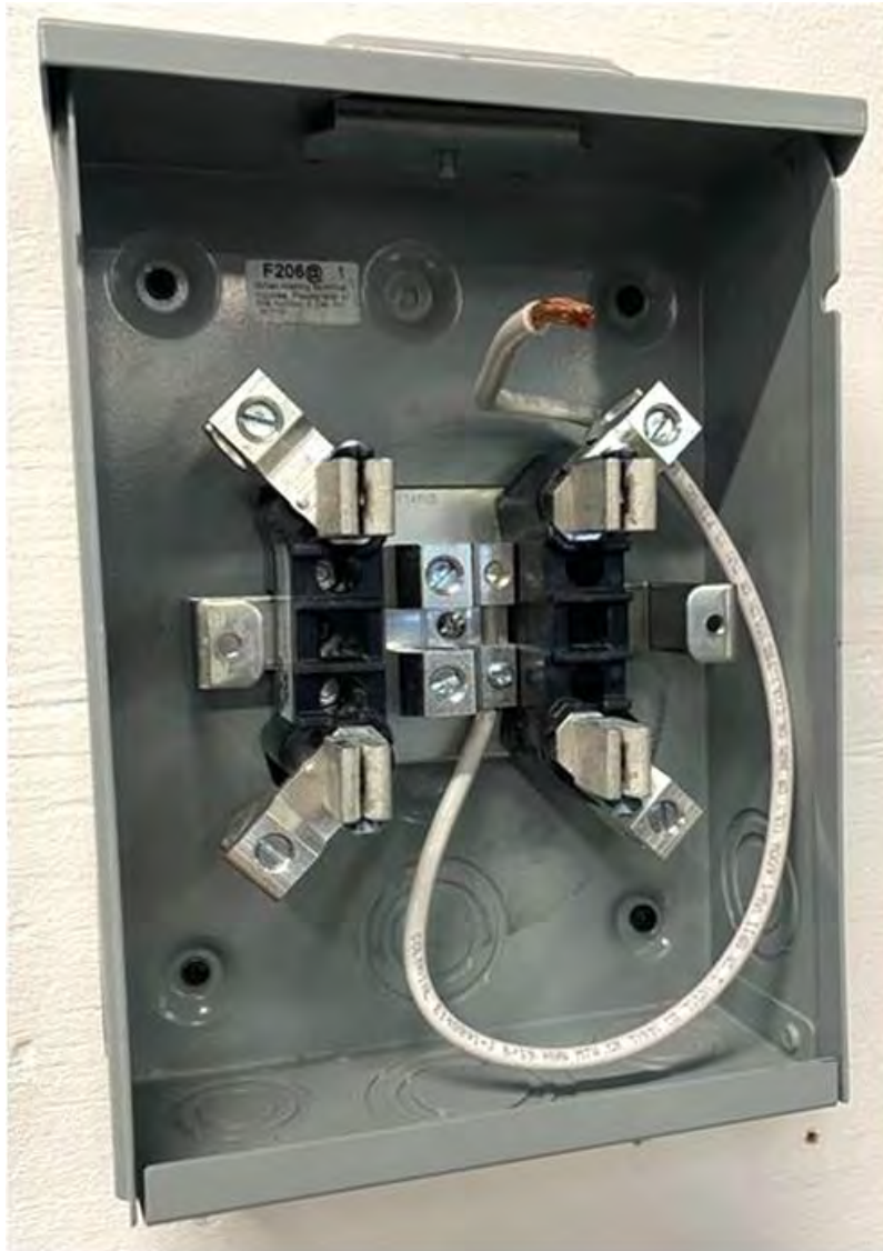
Figure 15 – Route the Neutral Within Meter Socket
