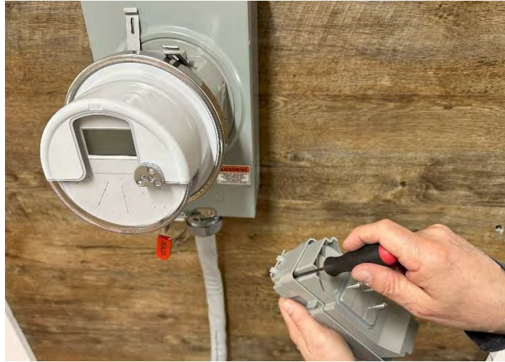
Figure 30 – Junction Box Removed.
