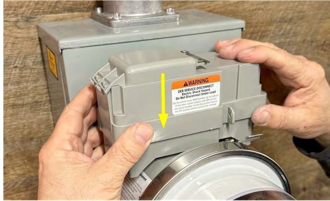
Figure 27 – Junction Box Installation
