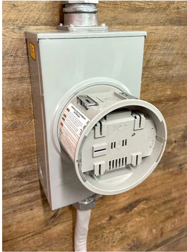
Figure 19 – Reinstall the Meter Socket Cover
