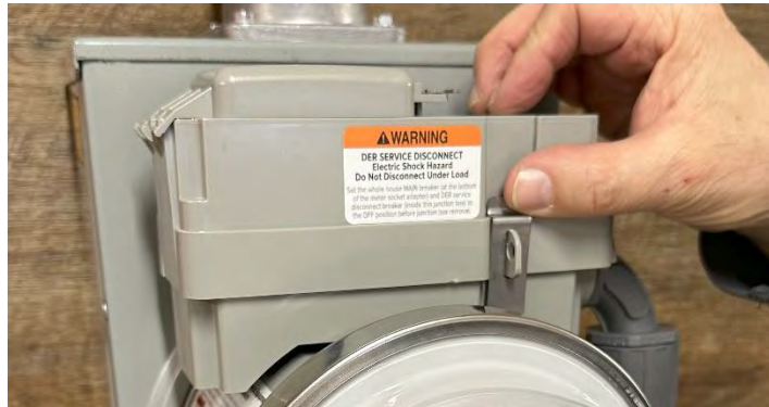
Figure 34 – Secure Junction Box Clasps
