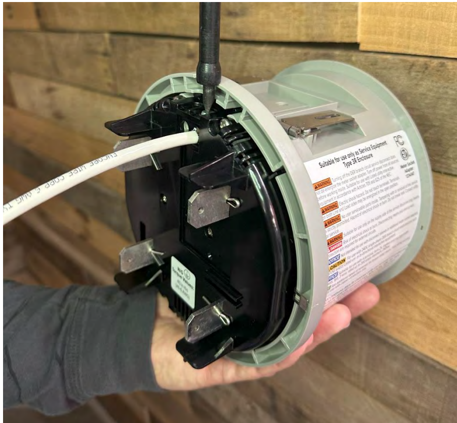
Figure 17 – Terminate the Neutral to the EV MSA
