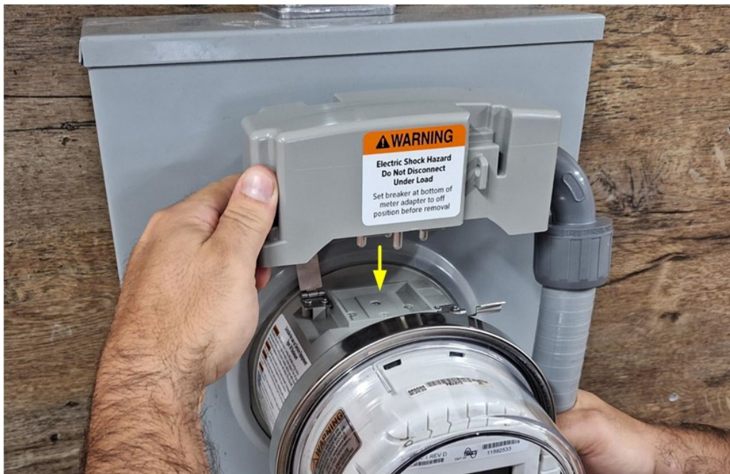
Figure 26 – Align the Junction Box Pins
