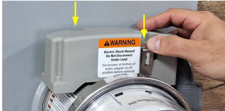
Figure 27 – Secure the Clasps
