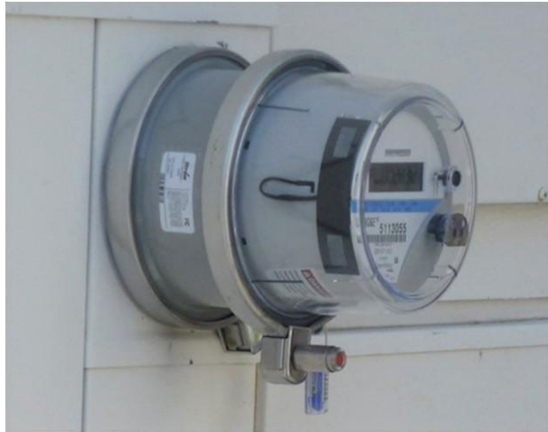
Figure 8 – Existing Meter and Socket Adapter
