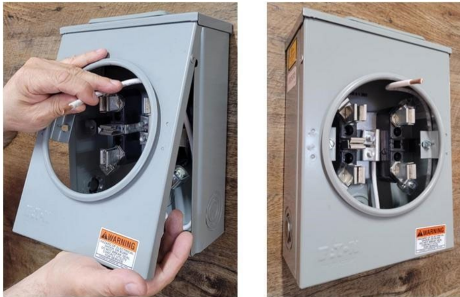
Figure 13 – Reinstall the Ring-Type Cover
