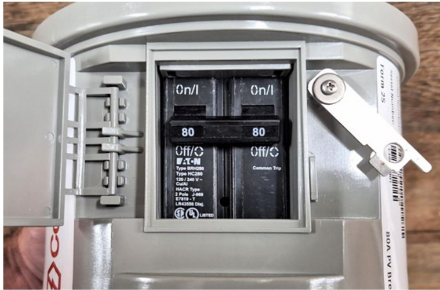
Figure 15 – Verify MSA circuit breaker is open (OFF)
