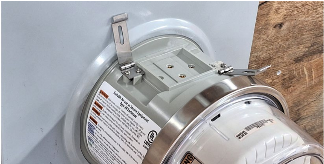
Figure 19 – Junction Box Locking Clasps
