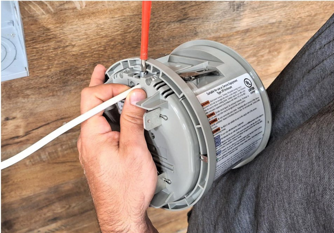
Figure 14 – Terminate the Neutral to MSA
