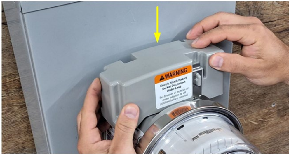
Figure 21 – Junction Box Installation
