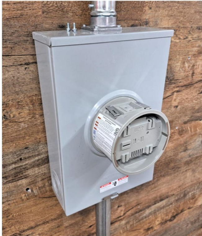
Figure 16 – Reinstall the Meter Socket Cover
