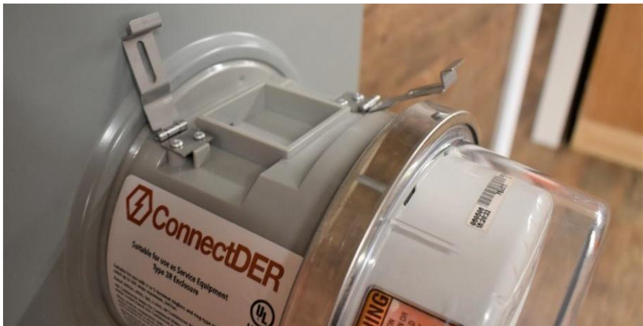
Figure 27 – Junction Box Locking Clasps
