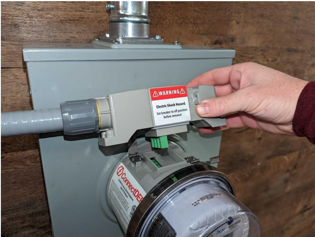
Figure 34 – Align the Junction Box Pins
