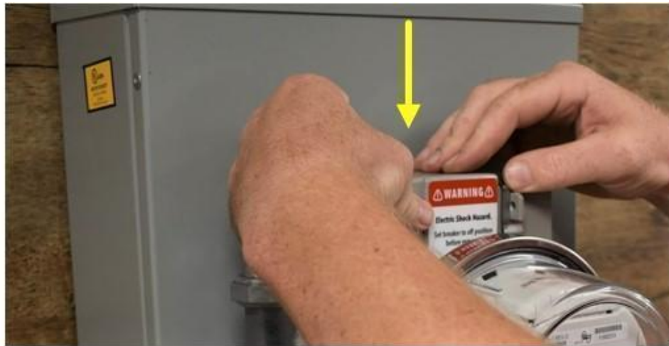
Figure 29 – Junction Box Installation
