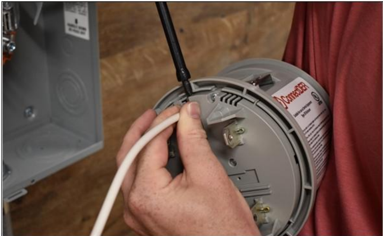
Figure 22 – Terminate the Neutral to Solar Meter Adapter
