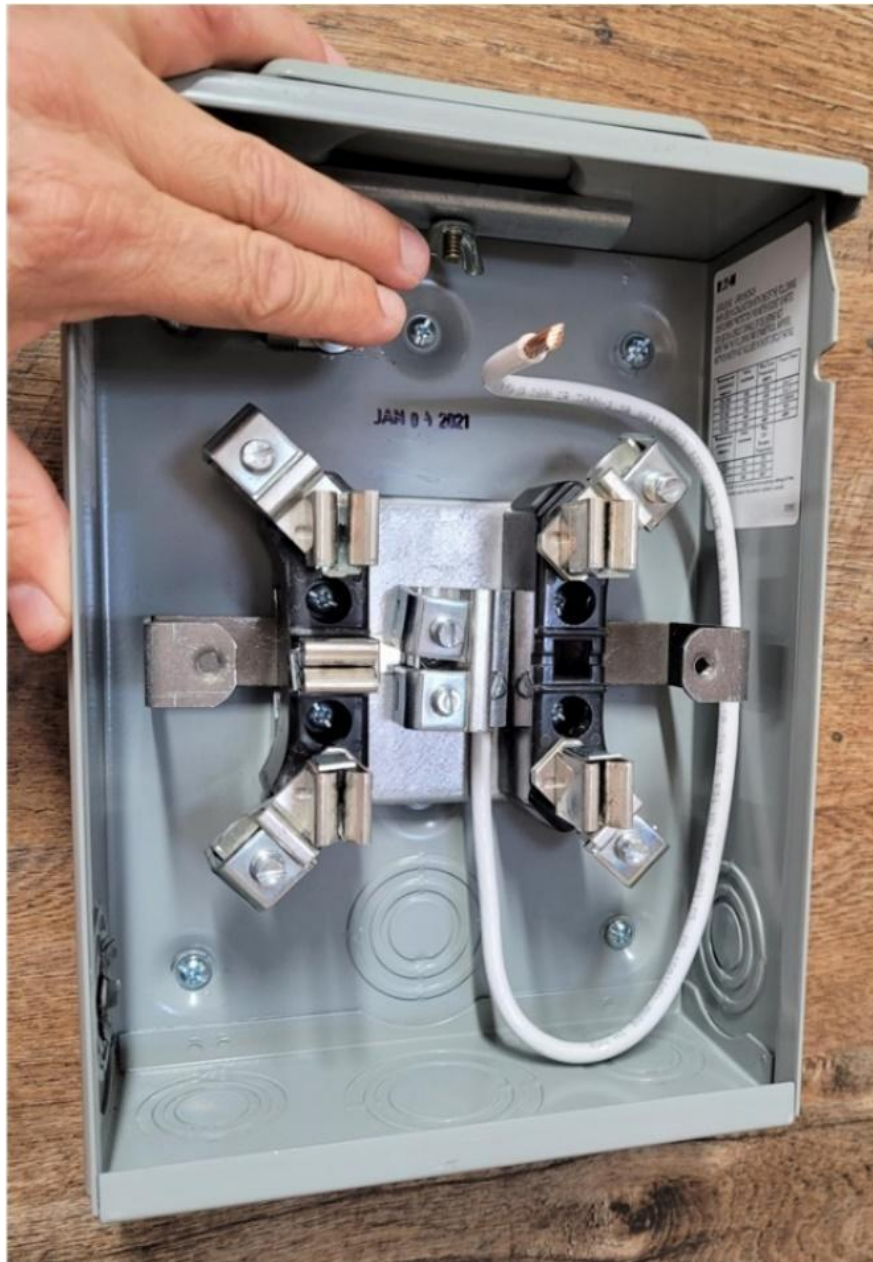
Figure 13 – Route the Neutral Within Meter Socket
