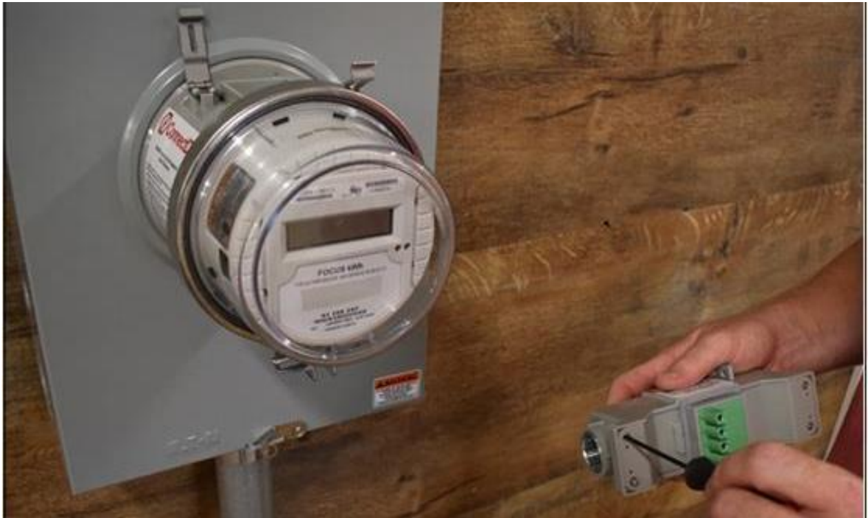
Figure 31 – Junction Box Removed
