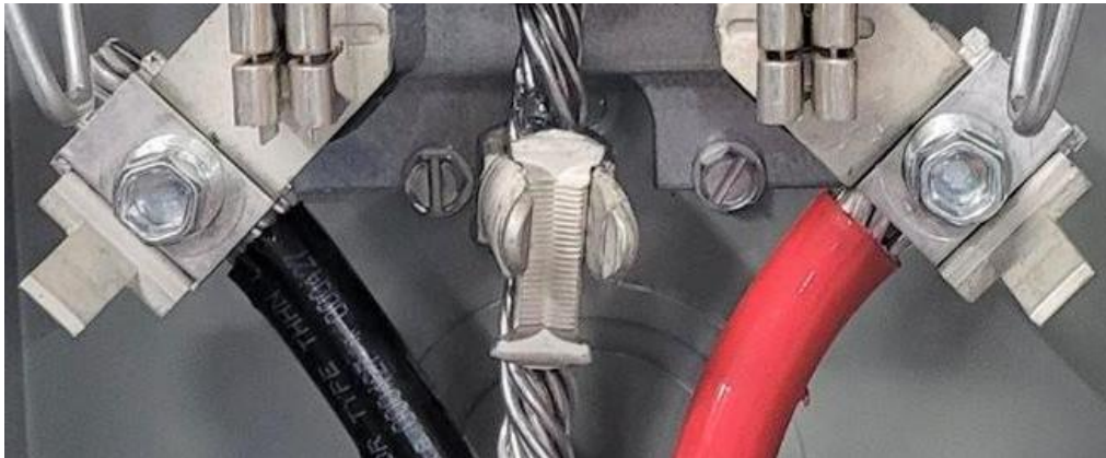
Figure 18 – Run and Tap Separator
