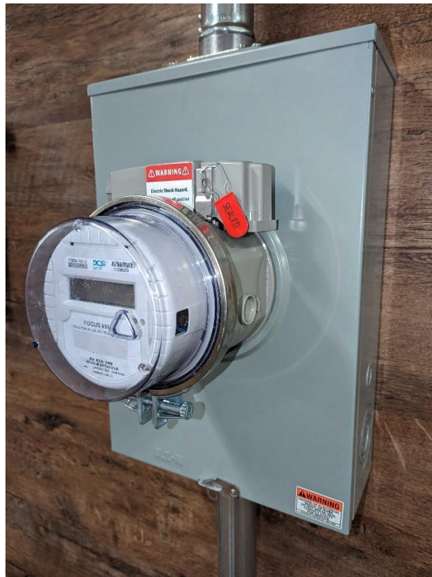
Figure 30 – Tamper-Prevention Seals
