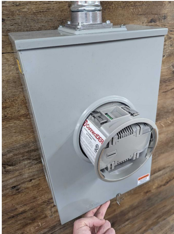
Figure 24 – Reinstall the Meter Socket Cover
