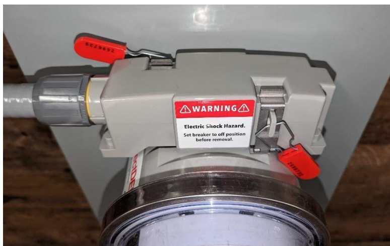
Figure 36– Tamper-Prevention Seals
