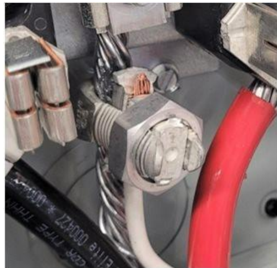
Figure 19 – Split-Bolt Connection
