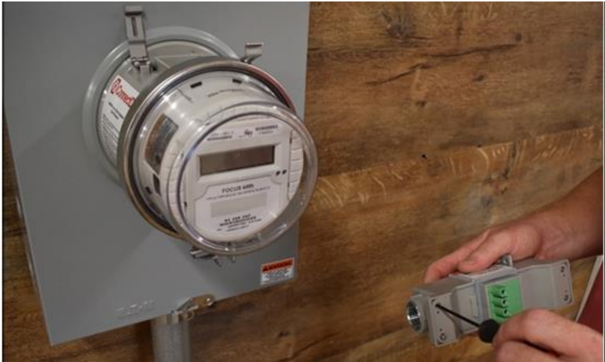
Figure 24 – Junction Box Removed
