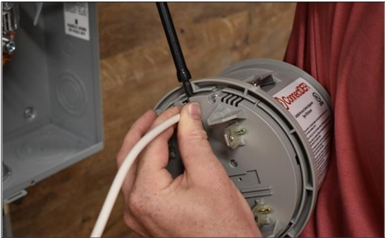
Figure 15 – Terminate the Neutral to MSA
