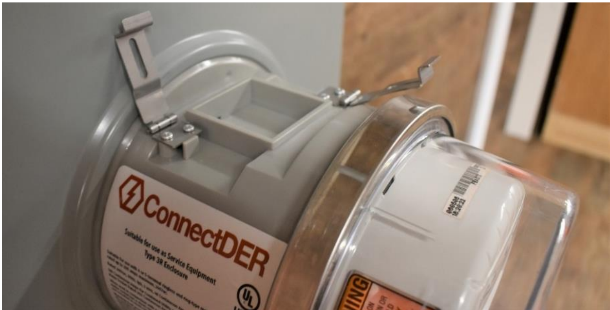
Figure 20 – Junction Box Locking Clasps
