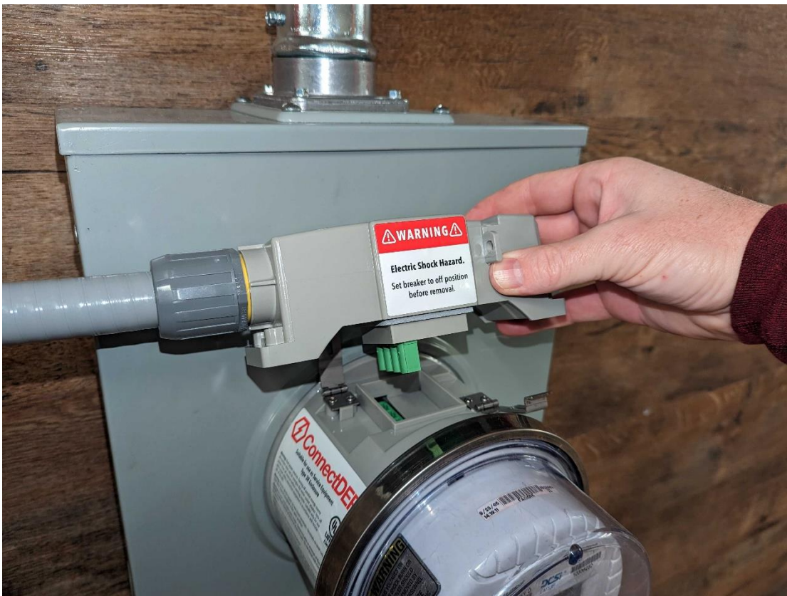
Figure 27 – Align the Junction Box Pins
