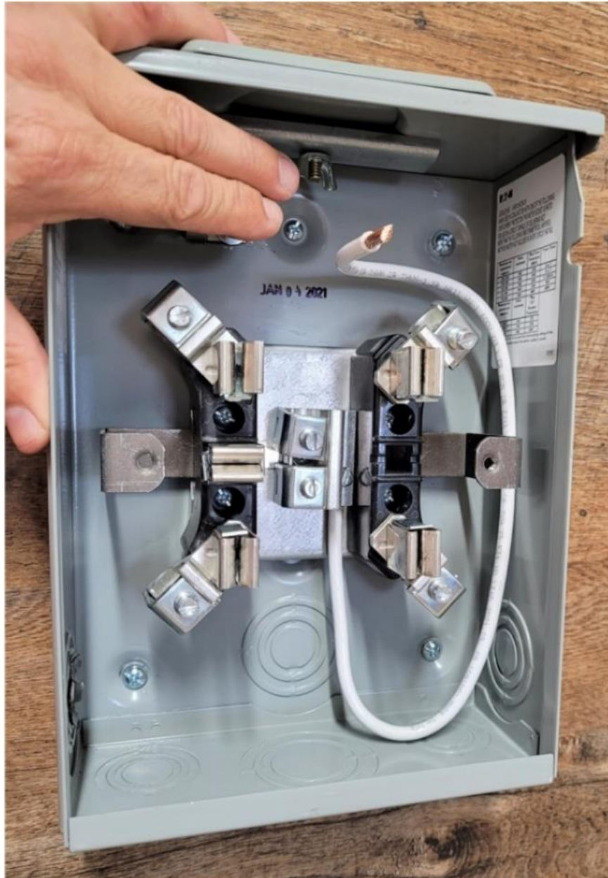
Figure 13 – Route the Neutral Within Meter Socket
