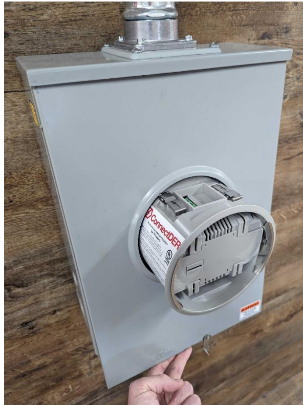
Figure 17 – Reinstall the Meter Socket Cover
