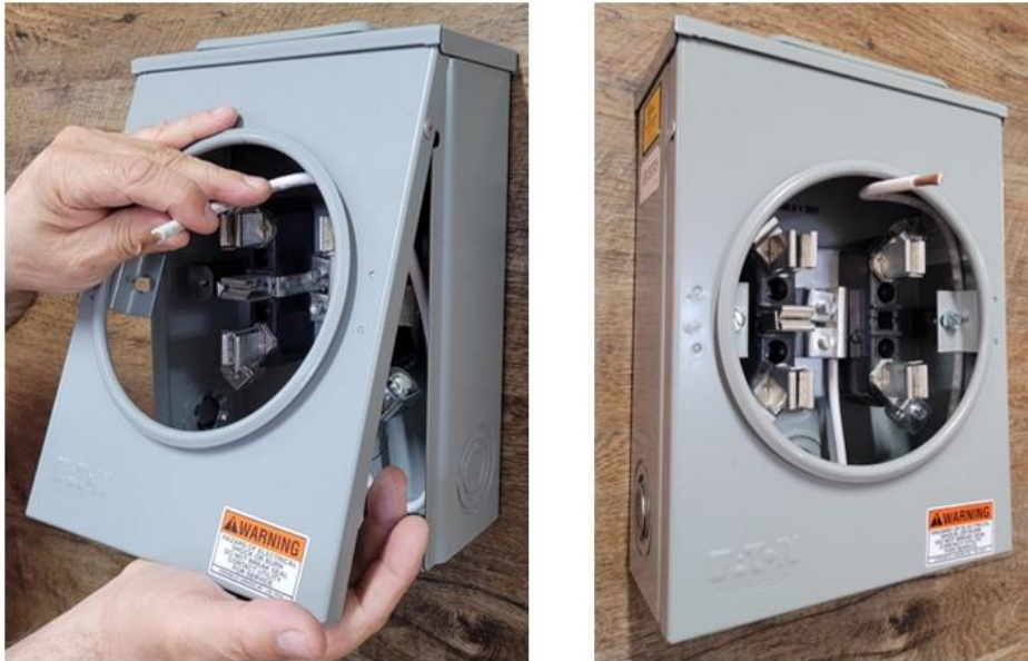
Figure 14 – Reinstall the Ring-Type Cover
