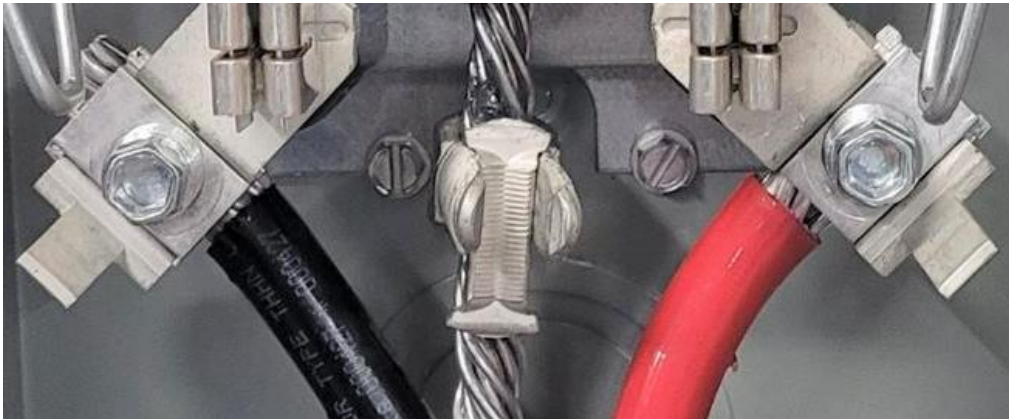
Figure 18 – Run and Tap Separator
