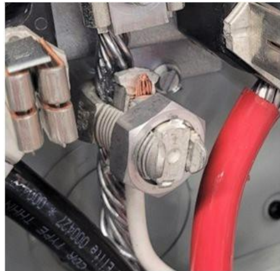
Figure 19 – Split-Bolt Connection
