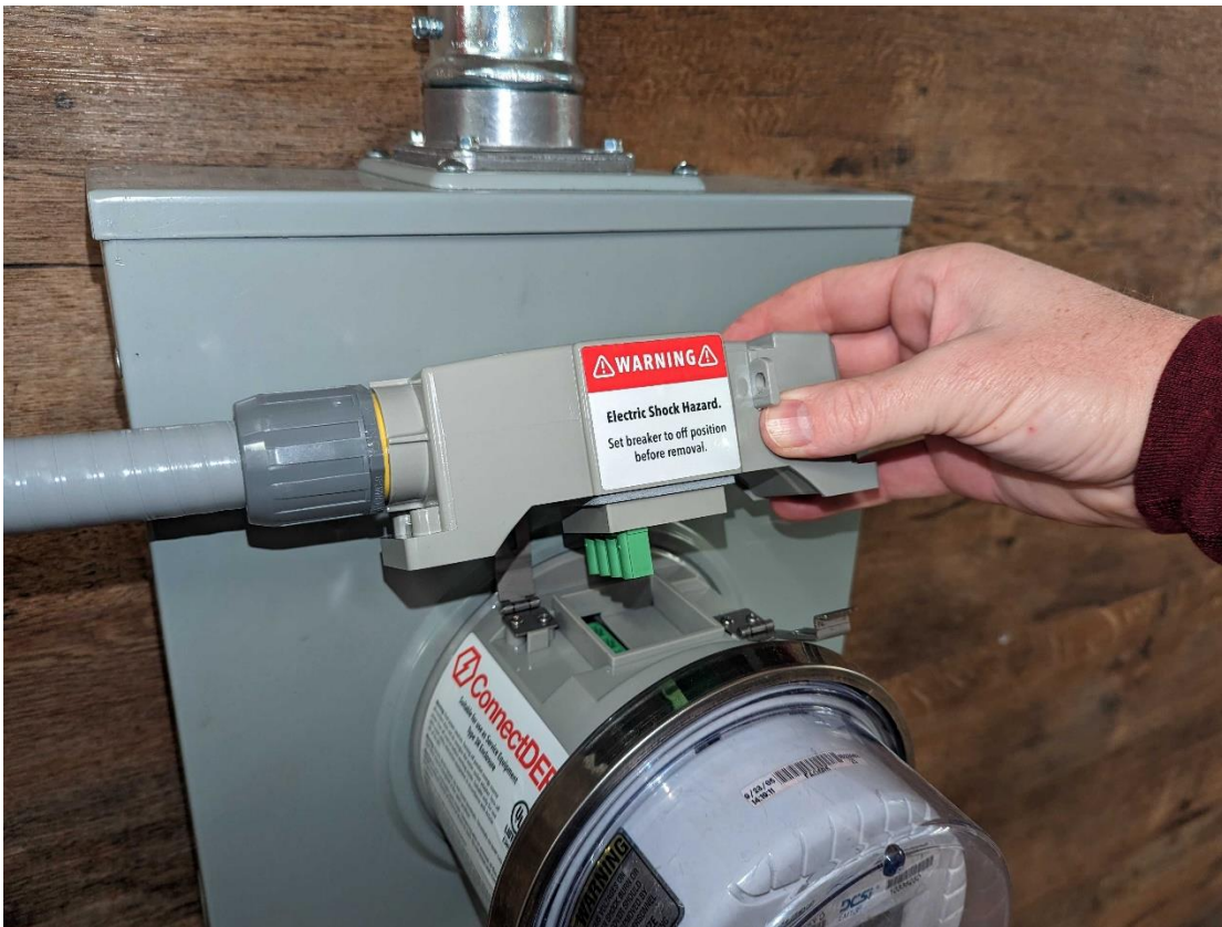
Figure 34 – Align the Junction Box Pins
