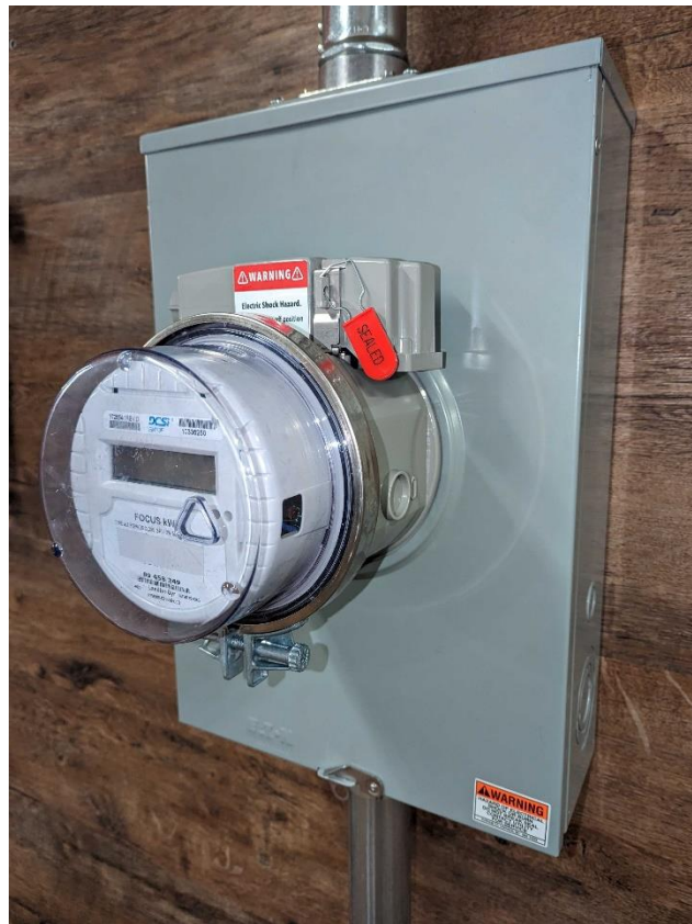
Figure 30 – Tamper-Prevention Seals
