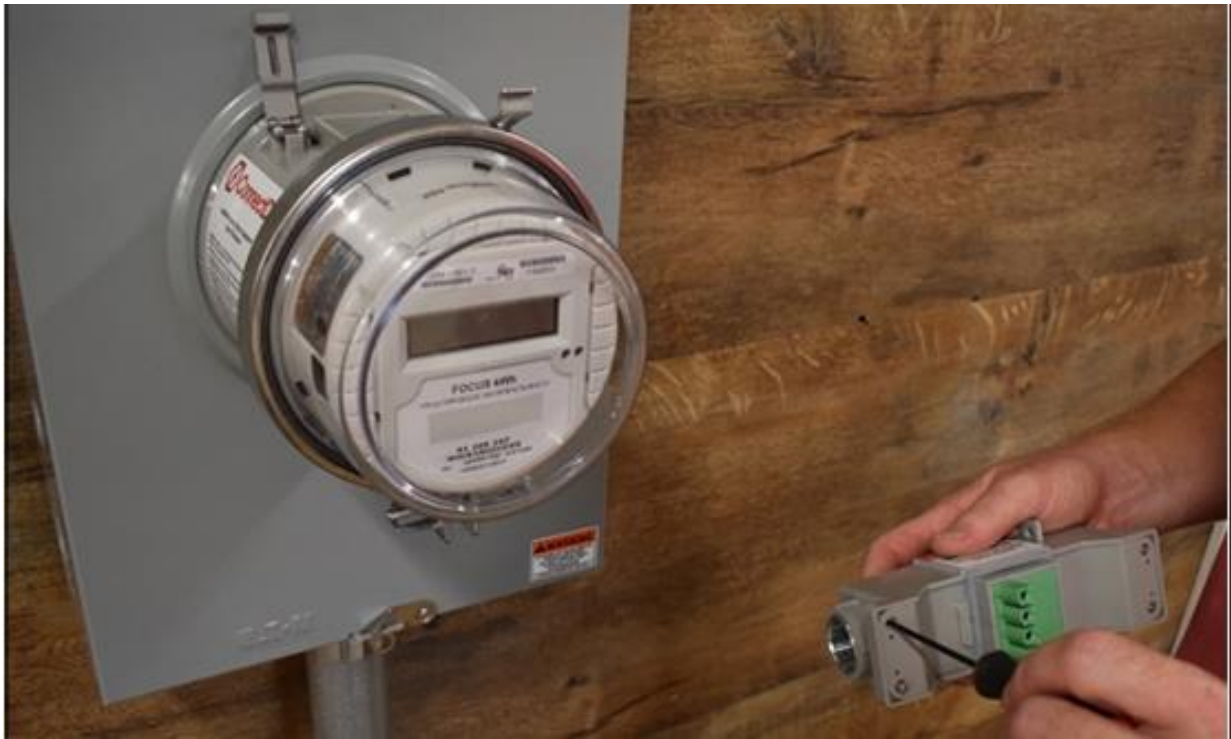
Figure 31 – Junction Box Removed
