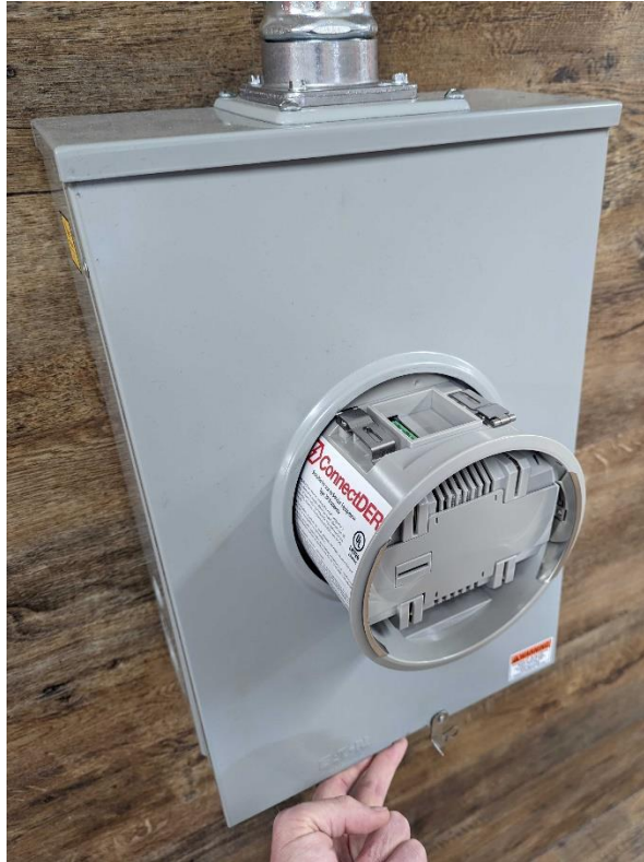
Figure 24 – Reinstall the Meter Socket Cover
