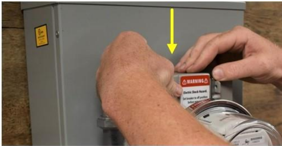
Figure 29 – Junction Box Installation
