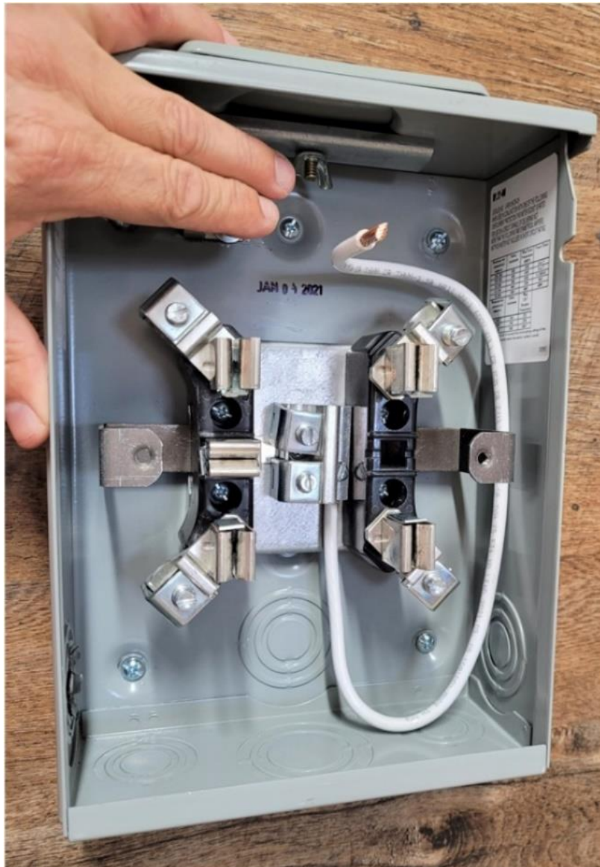
Figure 13 – Route the Neutral Within Meter Socket
