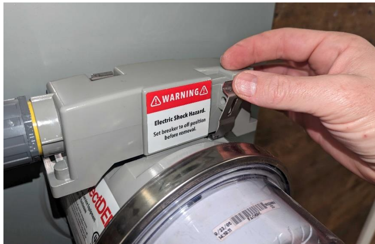
Figure 35 – Secure the Clasps
