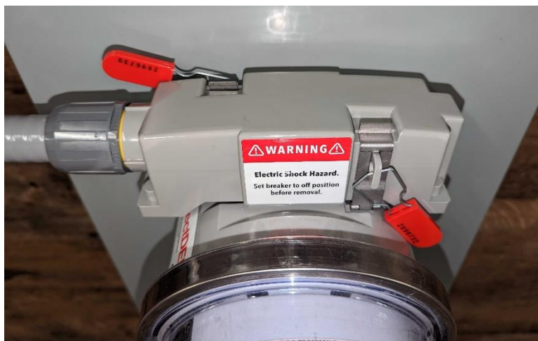
Figure 36– Tamper-Prevention Seals
