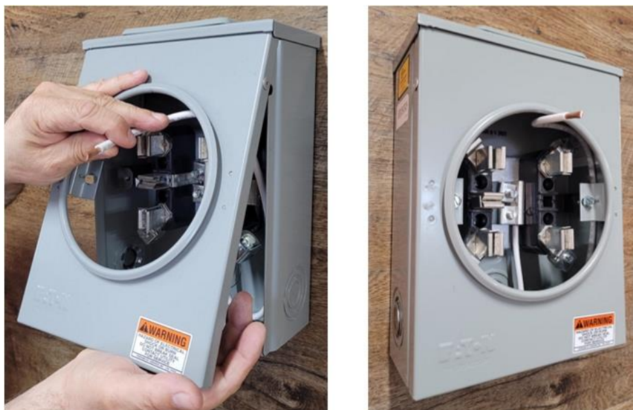
Figure 21 – Reinstall the Ring-Type Cover
