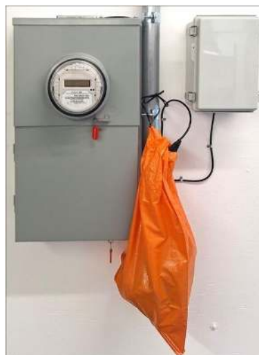
Figure 45. DER System Completed, Ready for MSA Installation.
