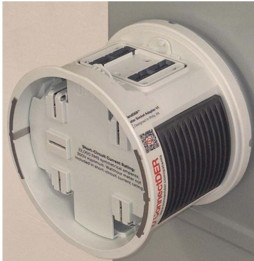
Figure 21. MSA Base Inserted in ringless socket.
