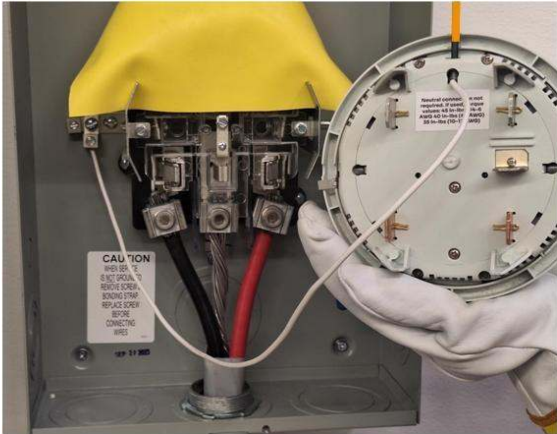
Figure 20. Field-Supplied Neutral Connection for Meter Sockets with 5 th Jaw at 6 o'clock.
