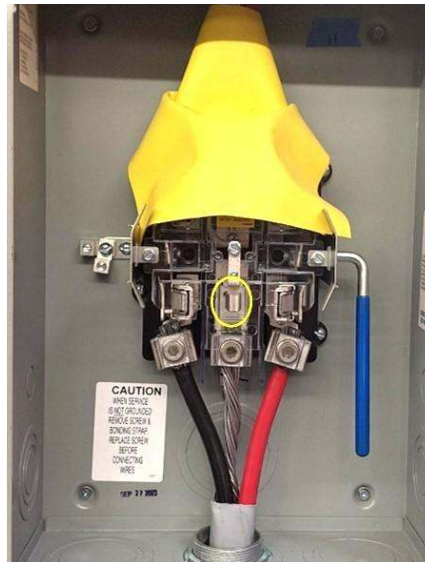
Figure 16. Protection From Energized Parts.
