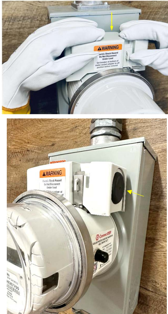
Figure 35. The MSA Connection Module is installed on top of the MSA Base. The clasps are closed and the black conduit entry hole closure plug remains in place (bottom image).
