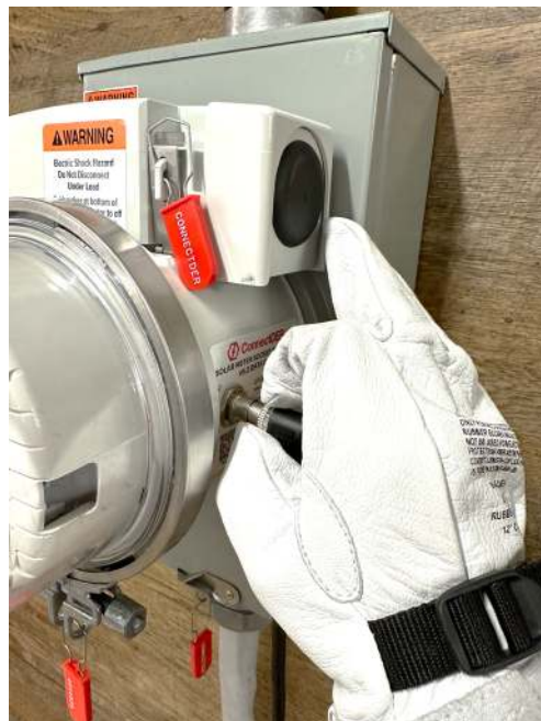
Figure 49. Once the CT Output Cable is on the CT Output Port, screw it in until it is secure.
