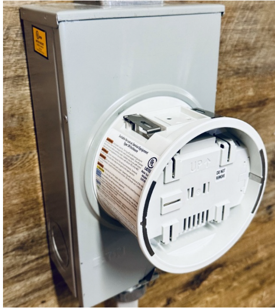
Figure 30. Reinstall the Meter Socket Cover.
