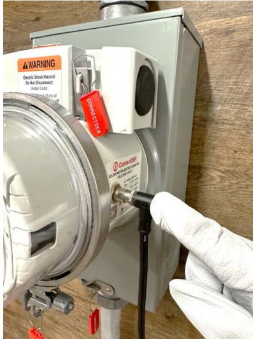
Figure 48. Make sure the CT Output Cable is fully seated in the CT Output Port before screwing it in.
