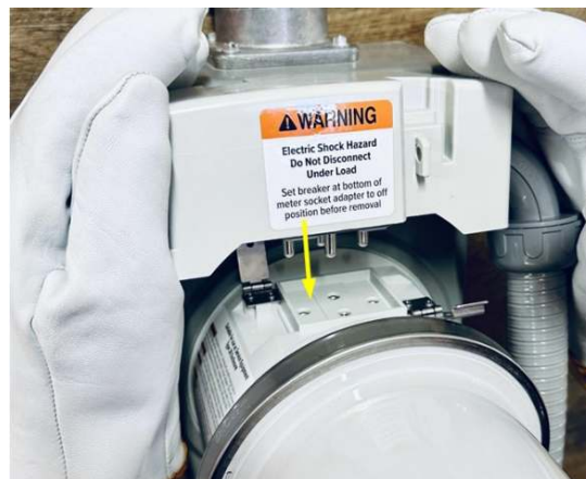
Figure 40. Align the Connection Module Pins over the Power Interface of the MSA Base.
