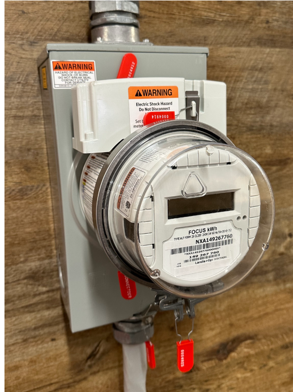
Figure 36. Tamper-Prevention Seals installed on the lock ring(s), Connection Modules clasps, meter socket, and the breaker cover on the bottom of the MSA Base.
