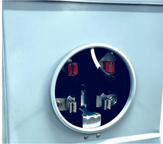
Figure 26. Reinstall the Ring-Type Cover.
