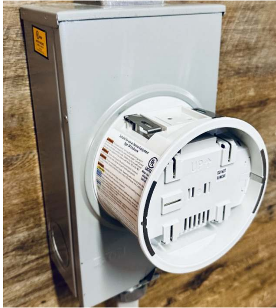
Figure 30. Reinstall the Meter Socket Cover.
