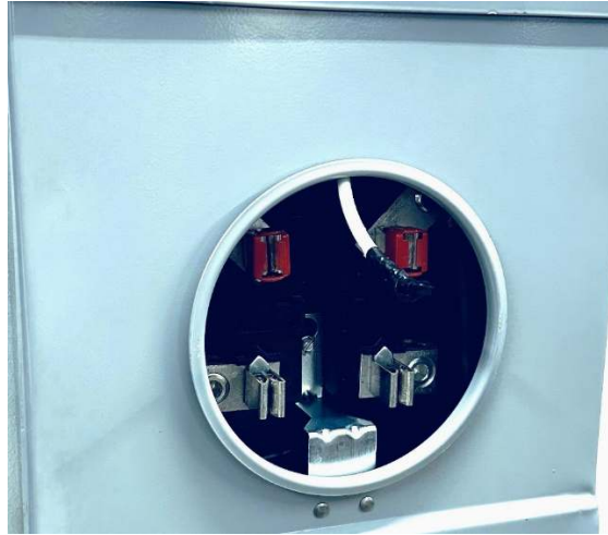
Figure 26. Reinstall the Ring-Type Cover.
