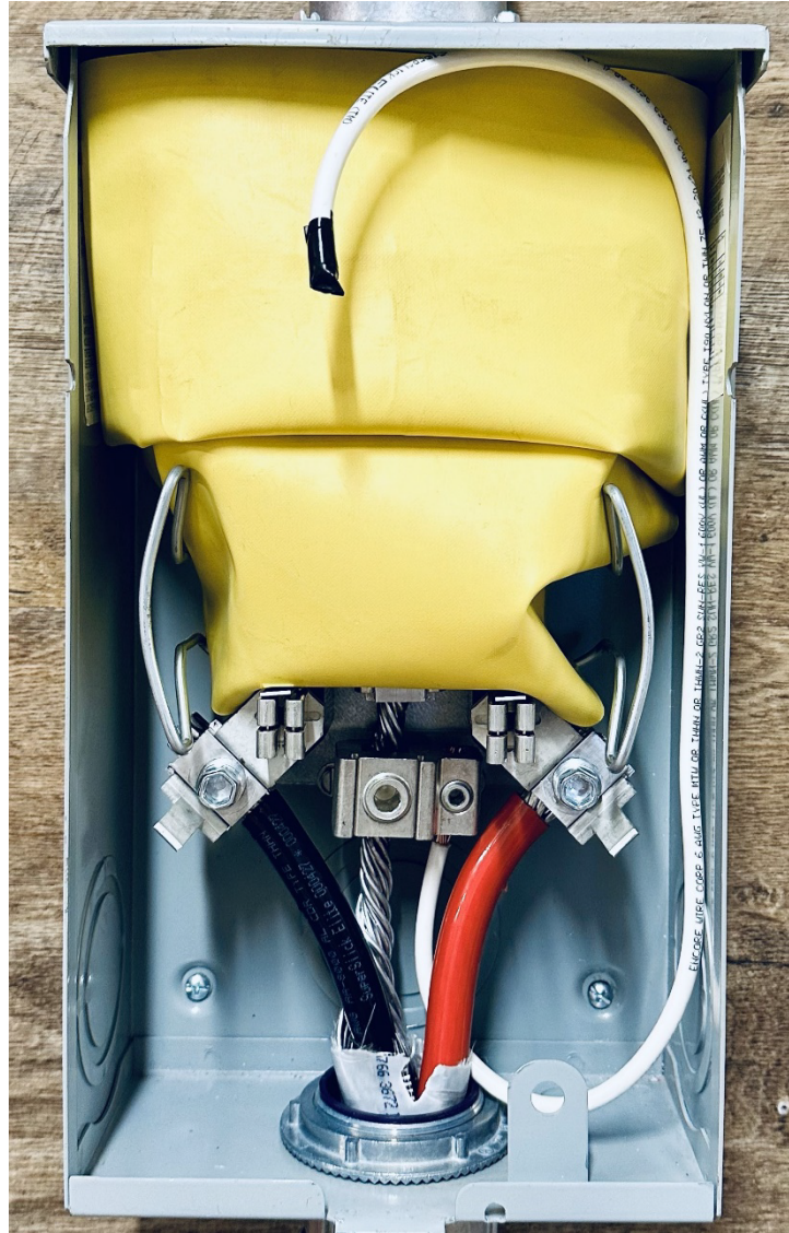
Figure 25. Route the Neutral Within Meter Socket.
