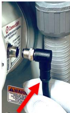
Figure 47. The CT Output Cable plugs in with the cable facing down.
