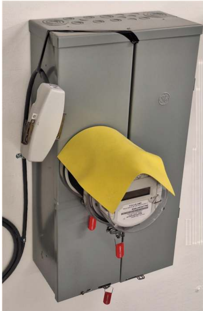
Figure 29. Connection Module Temporarily Supported, Communications Cable Deenergized, MSA Base Protected.
