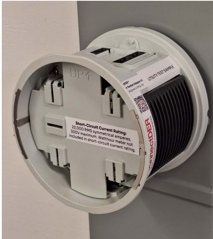
Figure 21. MSA Base Inserted in ring-type socket.
