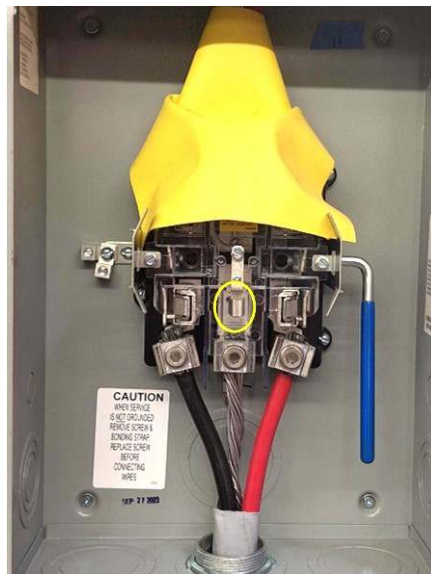
Figure 16. Protection From Energized Parts.
