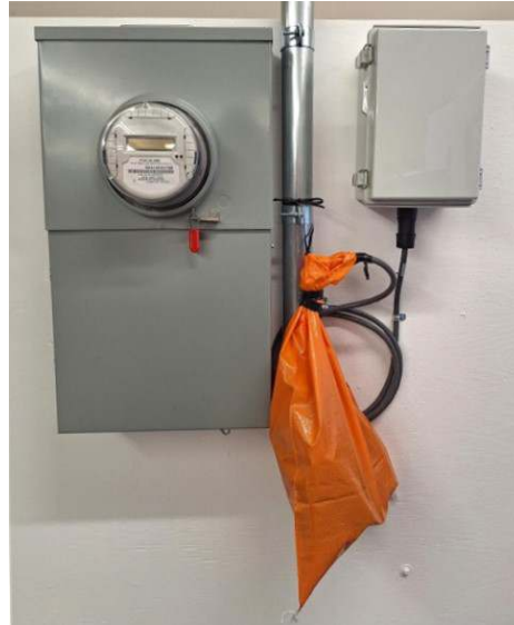
Figure 42. DER System Completed, Ready for MSA Installation
