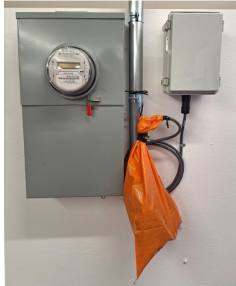
Figure 42. DER System Completed, Ready for MSA Installation
