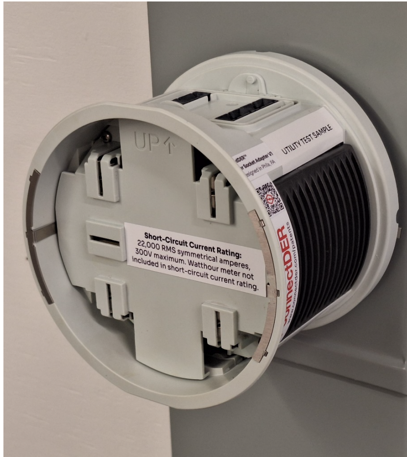
Figure 21. MSA Base Inserted in ring-type socket.
