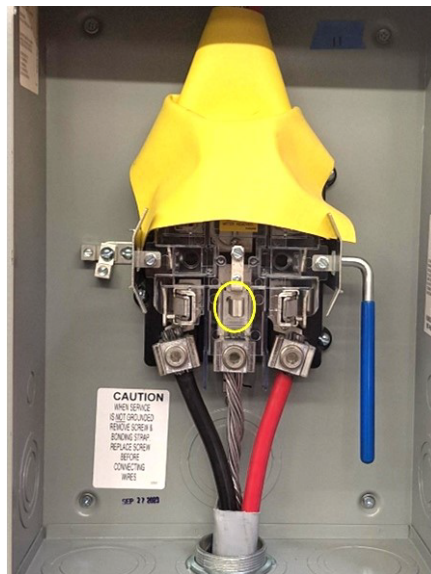
Figure 16. Protection From Energized Parts.
